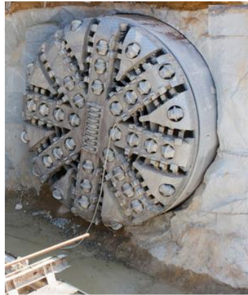
Figure 1. Tunneling boring machine
